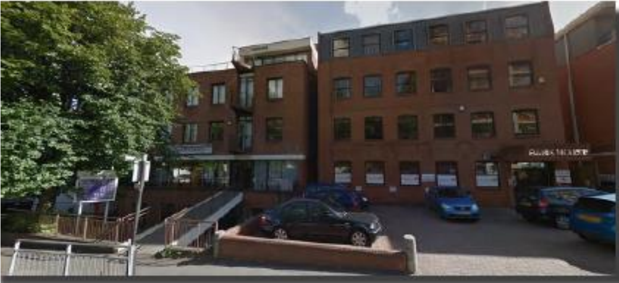
Front Elevation (Subject site to the left and Bank House to the right)
