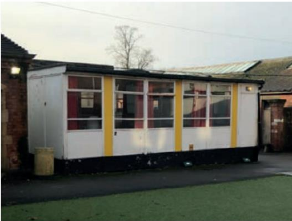
Portacabins to be demolished
