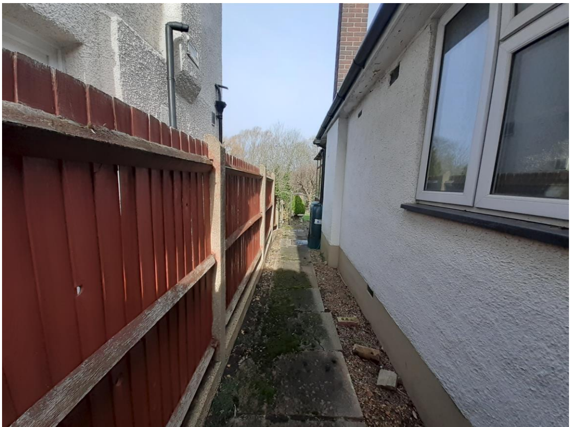
Northeast side access way, granting access from the front to the rear garden. Looking in the direction of the rear garden. No.44 over the fence to the left.
