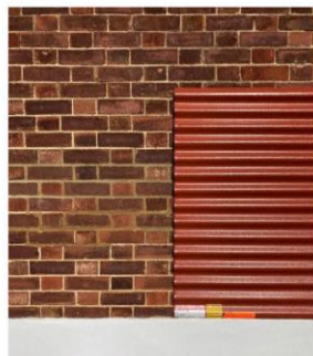
Figure 11 Boiler House with Proposed Cladding
