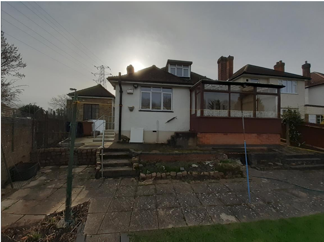
Rear elevation. Rear of existing garage (left). Existing conservatory (right).
