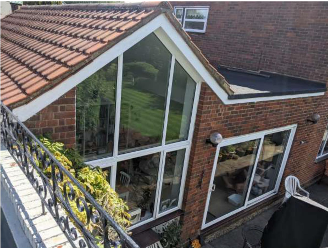
View of No. 9 Thornton Grove's Converted Garage
