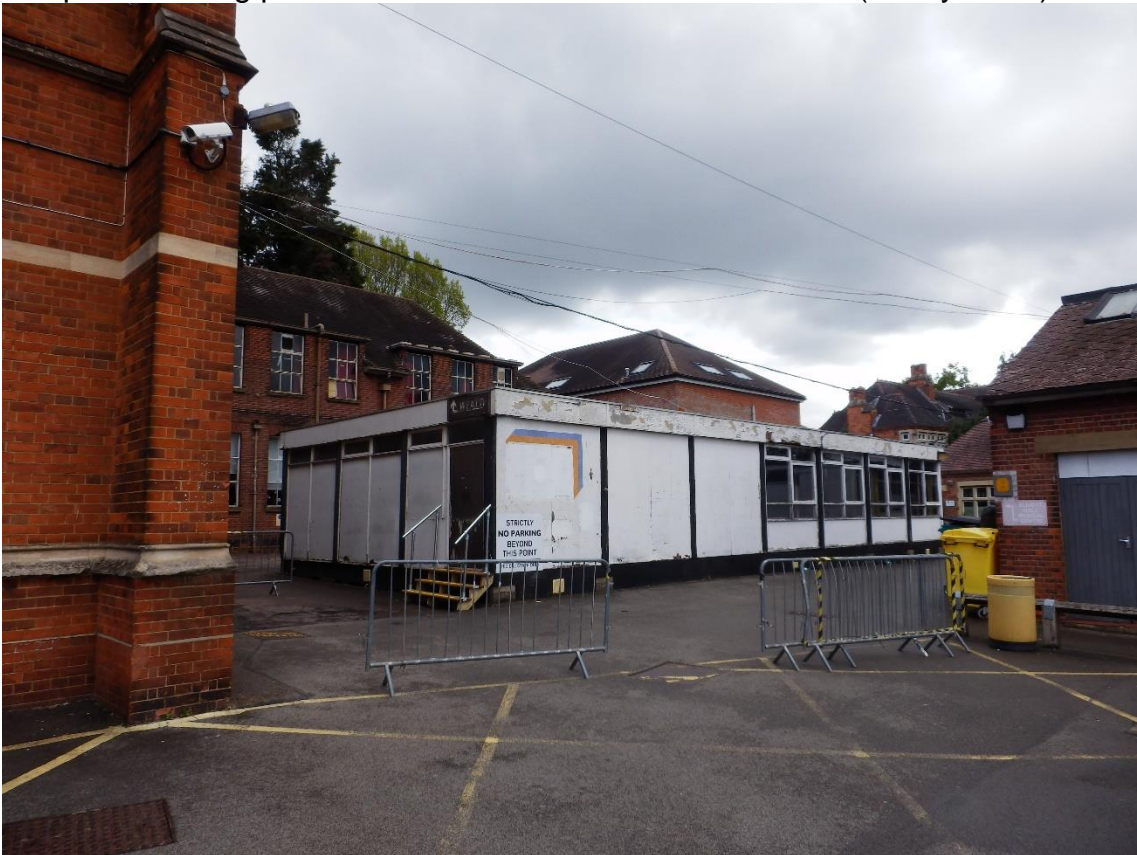
Portacabin to be demolished
