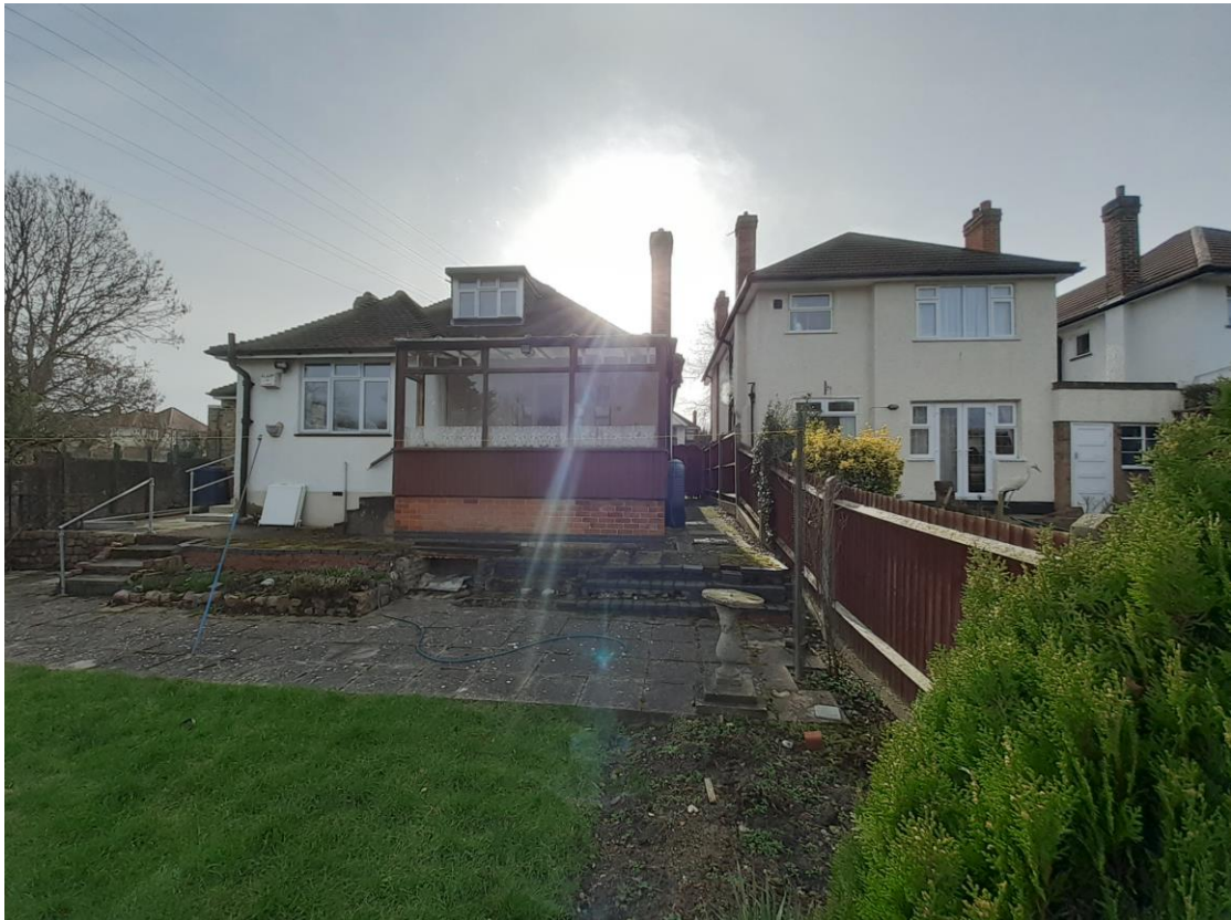
Rear view. Existing conservatory (centre). No.44 (right)
