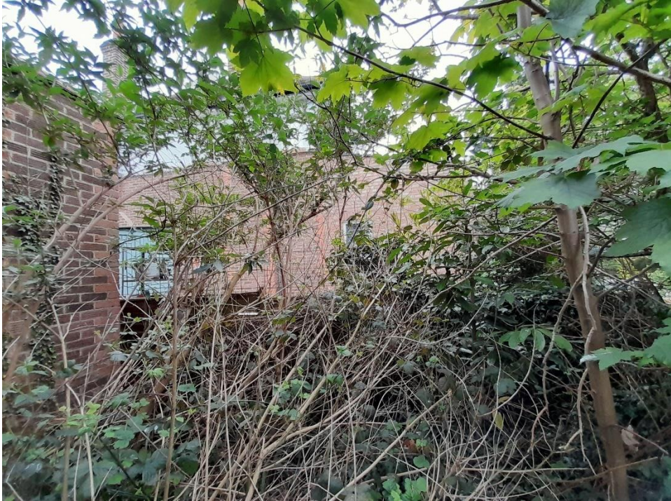
Side of No.19 and No.21
