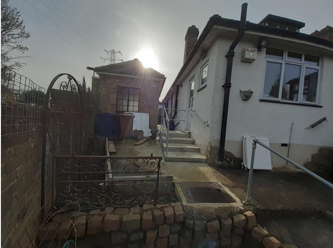
Southwest side access way, granting access from the front to the rear garden between the house and the garage.
